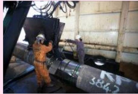
The last station is marine mastic station where the welded pipe joint is coated with hot marine mastic at a temperature of  $200 + 10^0$  C. The marine mastic will be fully poured into the mold which is wrapped around the pipe joints. Then the mold will be sealed and water cured.
