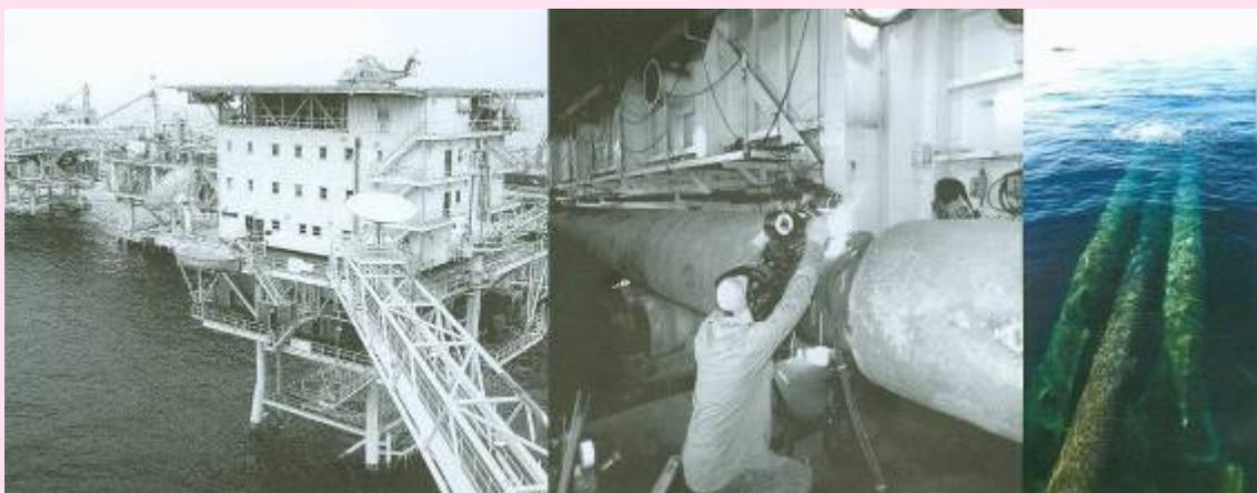
The pipes laid into the sea which forms S curve or S lay is designed to withstand both overbend and sagband stress.
