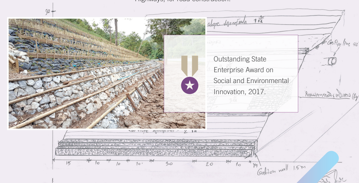
Vetiver grass implant in bamboo tubes.
