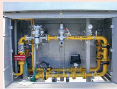
Metering and Regulating Station
